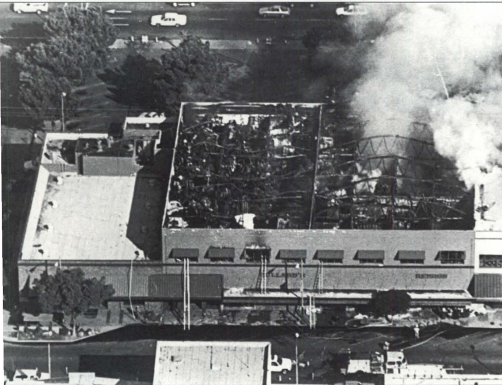
Bank of the Sierra's downtown Porterville (California) location lies in ruins following an October 2 fire.
